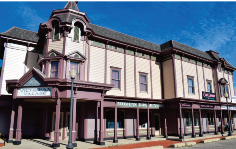
Victorian Village on Main Street, owned by Kraig Hardcastle, got a fresh paint job thanks to a façade improvement grant received in 2025.
