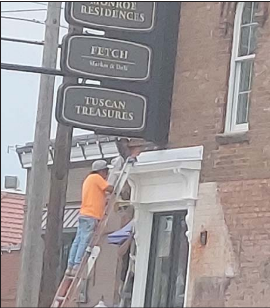
A worker paints the facade in front of 101 Monroe
