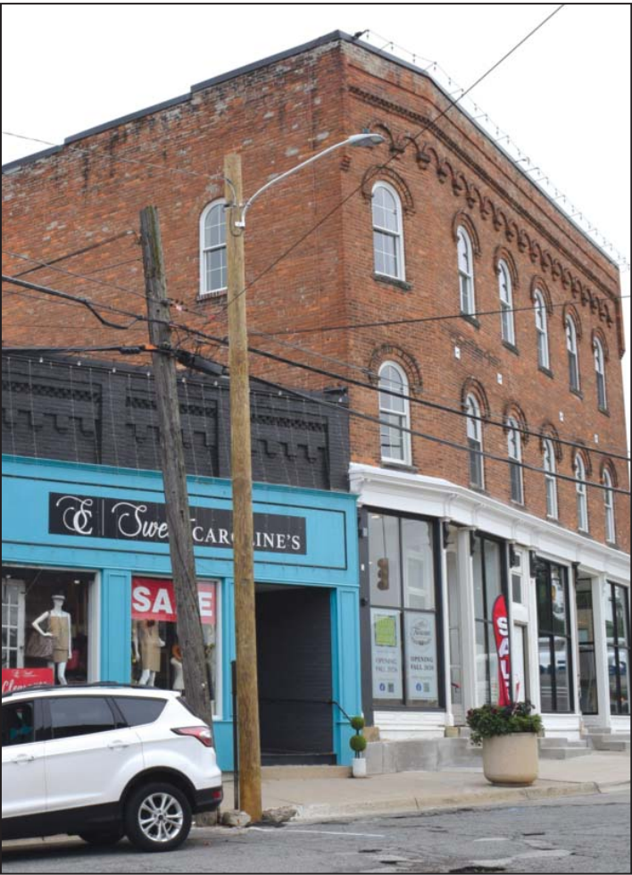
Construction at the corner of M-50 and Monroe street has caused some business owners to complain that it has hurt their bottom line, while others say tax credits the owner received for the building project are not fair.
