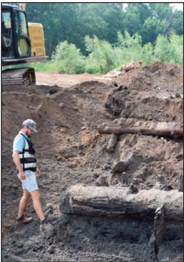
A construction worker toes the former dam, which was once made of logs, before Henry Ford bottled the River Raisin waterway with concrete.
