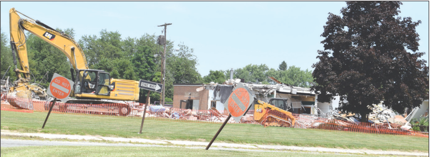
The former Ackerson Lake High School was reduced to rubble last week. Oscar Herrera of Handy Excavating LLC used the backhoe to raze the former high school.
