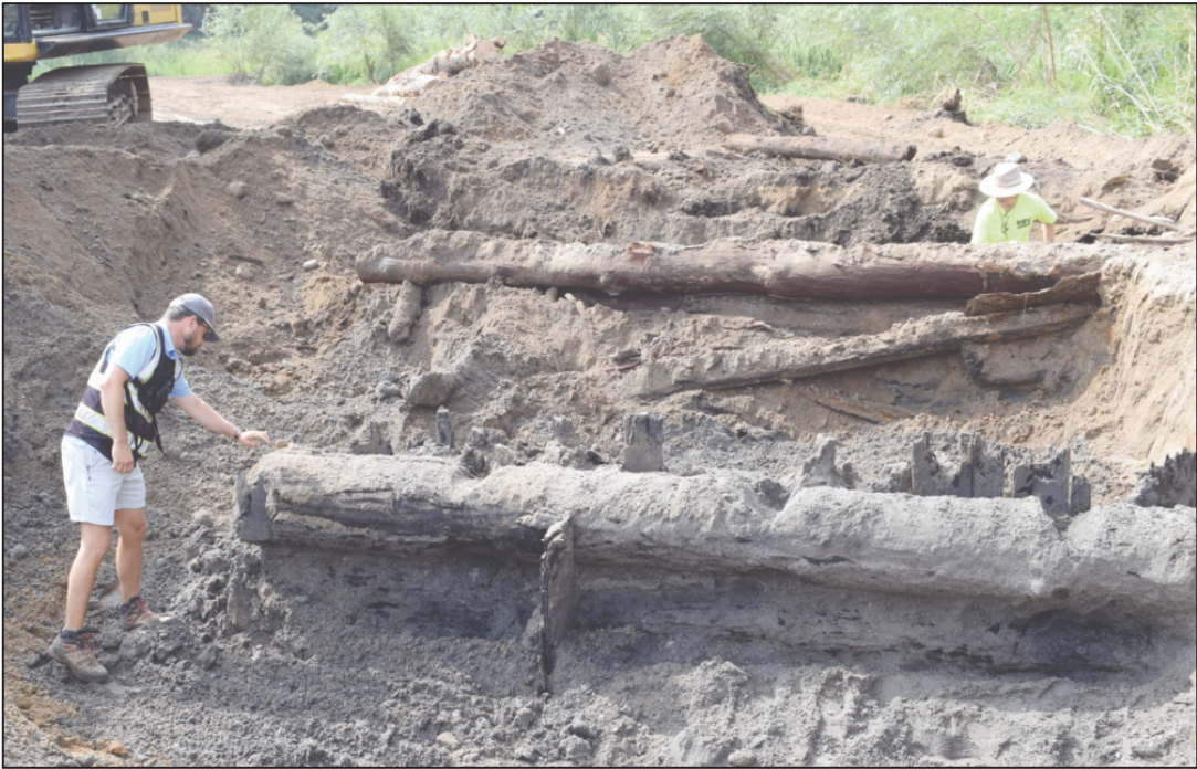
Riley Lecka, a heavy equipment operator for Wildlands Construction, points out the hand-hewed log that was used as part of a dam or spillway before 1938. Note the notches in the top of the log, which likely had something to do with controlling the water levels.
