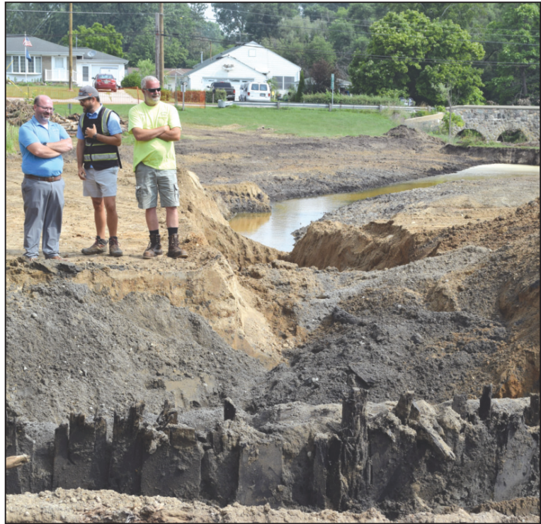
Village of Brooklyn Manager Matt Swartzlander, left, Riley Lecka of Wildlands Construction, and Dennis Spittler, Village of Brooklyn DPW Supervisor, discuss the ongoing construction project at the former mill pond site.
